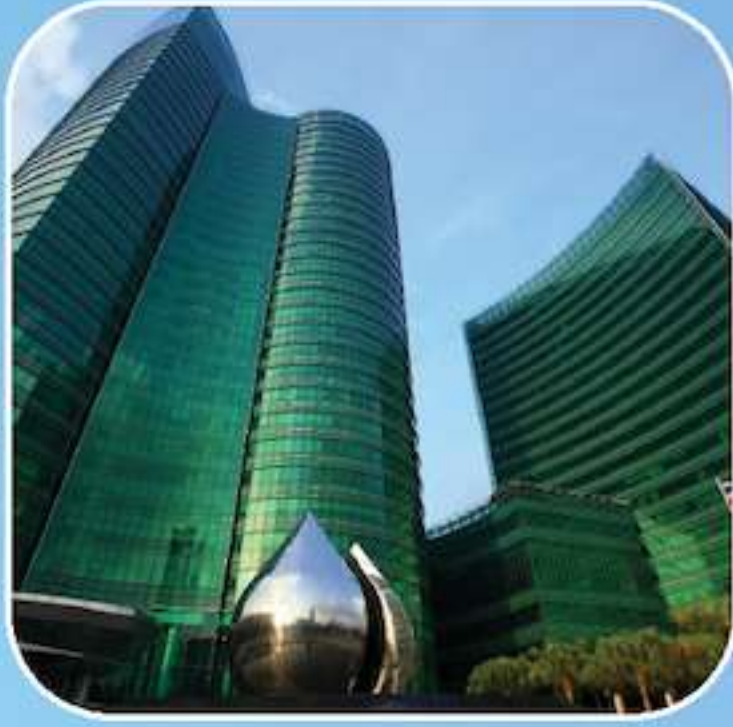
Energy Complex / PTT Head office, Chatuchak
